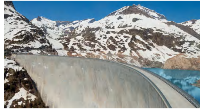
Staumauer Emosson (VS)
